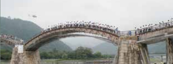
【The Strength Test (August 12, 2009)】 This is to check the safety of the bridge by measuring “how the bridge transforms when there are people on it”.
